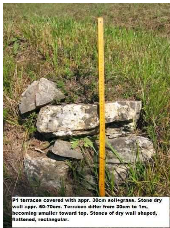
P1 terraces covered with soil and grass, built from dry walls, approx. height 60-70 cm. Rectangular stone slabs shaped to form dry wall. Foto G.Lukacs 2007
